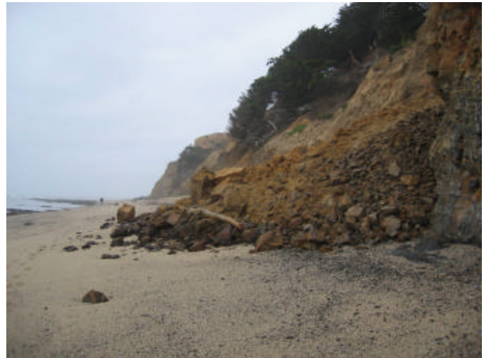
Figure 1-10. Recent landslide onto Moss Beach.
