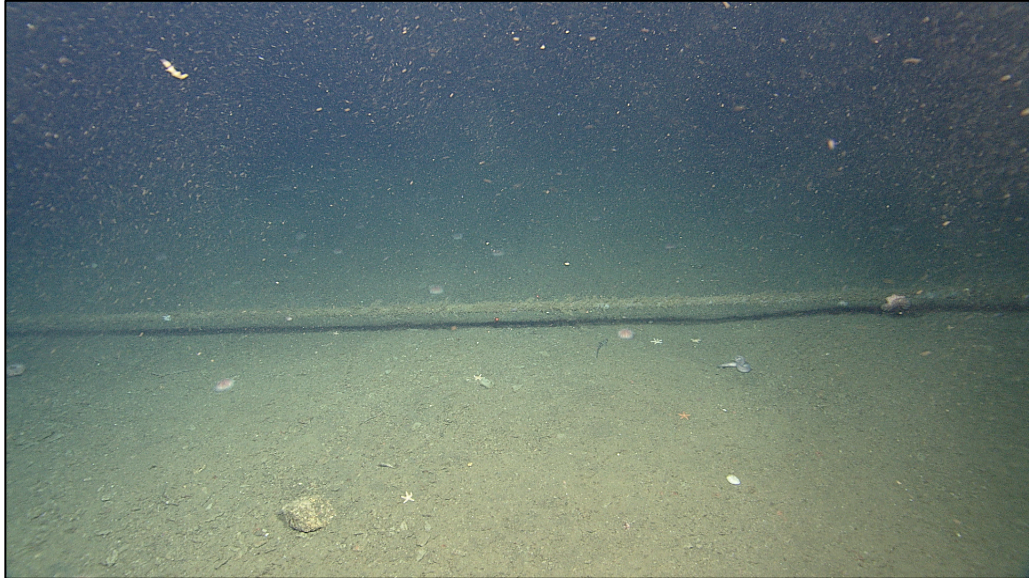
Figure I. Typical minor span where rocks or ledges prevent the cable from resting on the seafloor (316 m depth).
