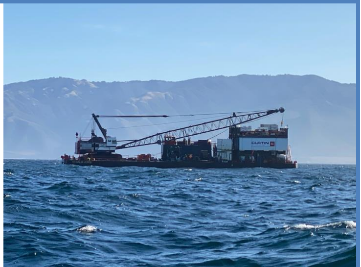
A large barge served as an operations platform to crane, ROV and dive teams to attempt salvaging of a sunken yacht of the Big Sur Coast. Photo Credit: B.Hoover, MBNMS
